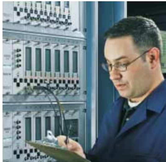
Cooper Compression's test center control room provides computer control of cooling water, input speed and lubricating oil supply.
